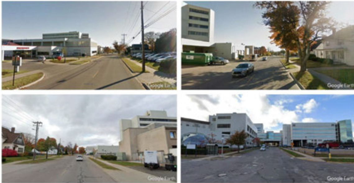
EXISTING CONDITIONS: FORMER MARQUETTE GENERAL HOSPITAL STRUCTURES
