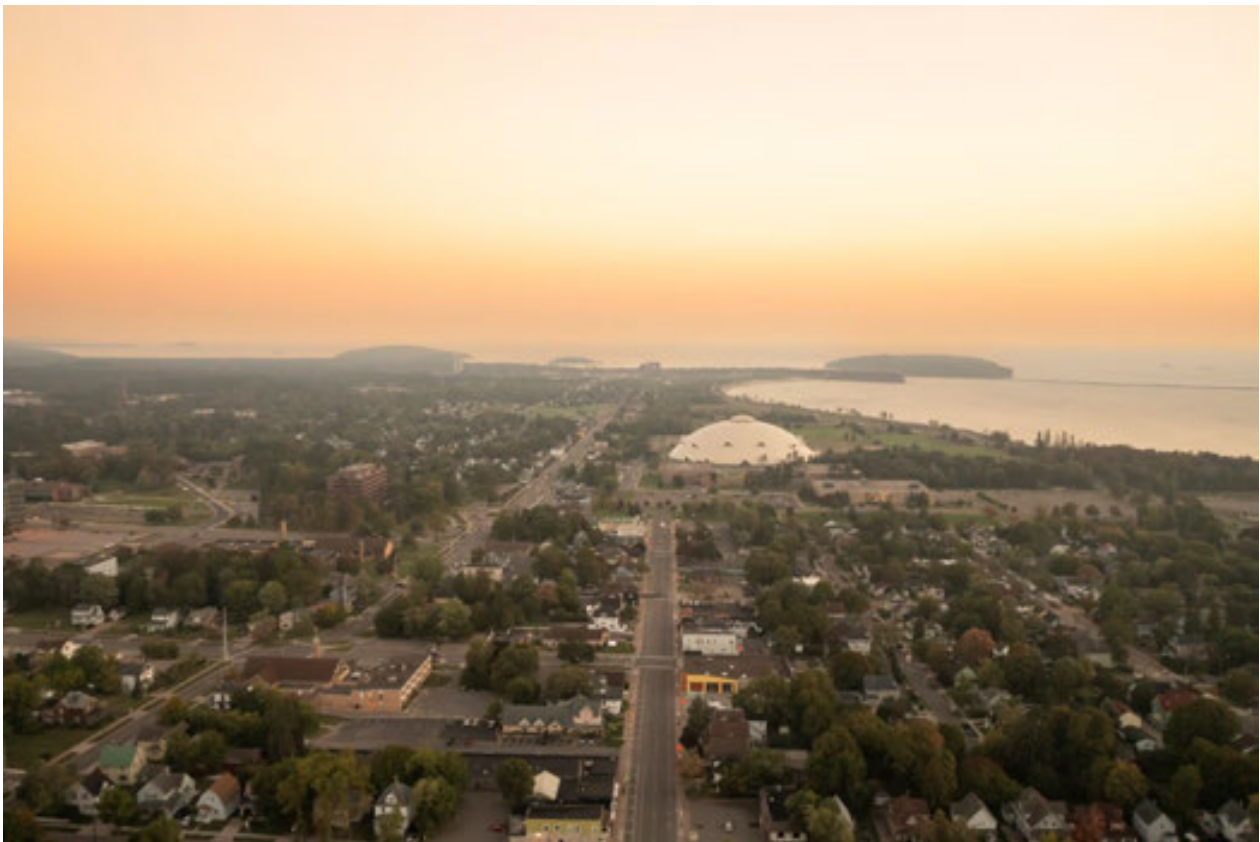
View of north Marquette and 3 rd Street business corridor. The eastern boundary of the site partially visible in the left.
