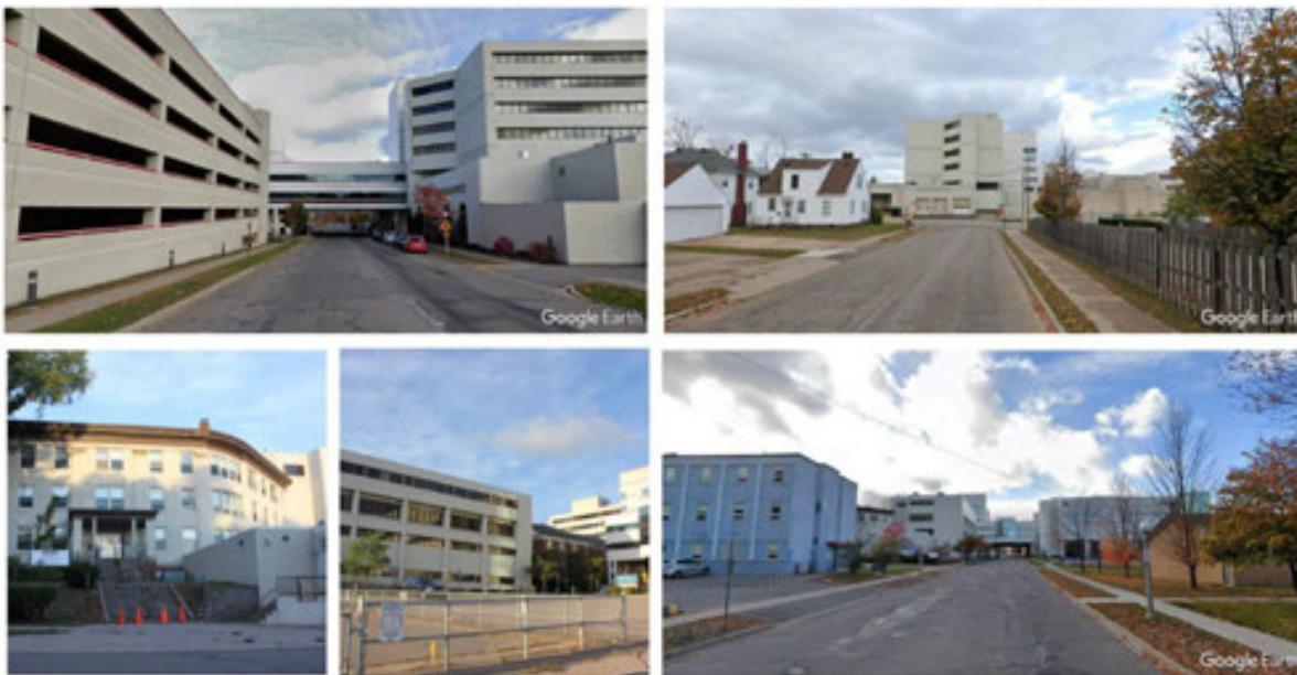
EXISTING CONDITIONS: FORMER MARQUETTE GENERAL HOSPITAL STRUCTURES
